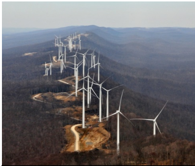
Figure 1: Wind turbines along a mountain ridge.
